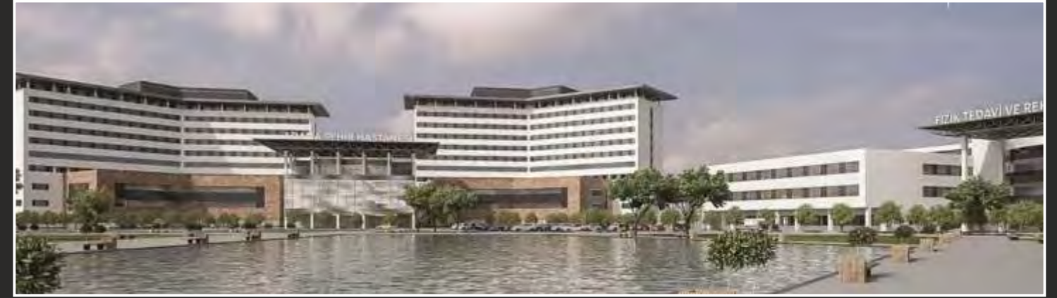
ADANA ŞEHİR HASTANESİ ADANA CITY HOSPITAL YATAK KAPASİTESİ 1550 BED CAPACITY 1550
